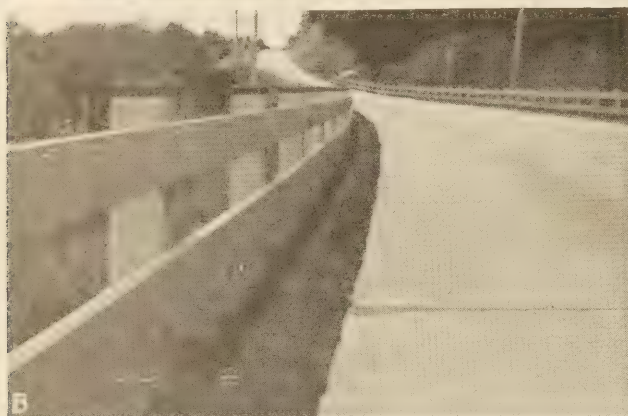
A, FIREBREAK STRIP FORMED BY TREATING VEGETATION WITH SODIUM CHLORATE. B, APPEARANCE DURING THE SUMMER OF AREA AROUND GUARDRAIL WHERE SODIUM CHLORATE WAS SPRAYED THE PREVIOUS FALL.
